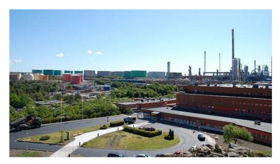
Preem is responsible for 80 percent of Swedish refinery capacity and 30 percent of Nordic capacity. In Preemraff Göteborg, Preem's biorefinery in West Sweden, crude tall diesel is converted into renewable diesel that comprises hydrocarbon equivalent to that in fossil diesel. It is then processed together with fossil raw materials to produce a diesel with renewable ingredients.
